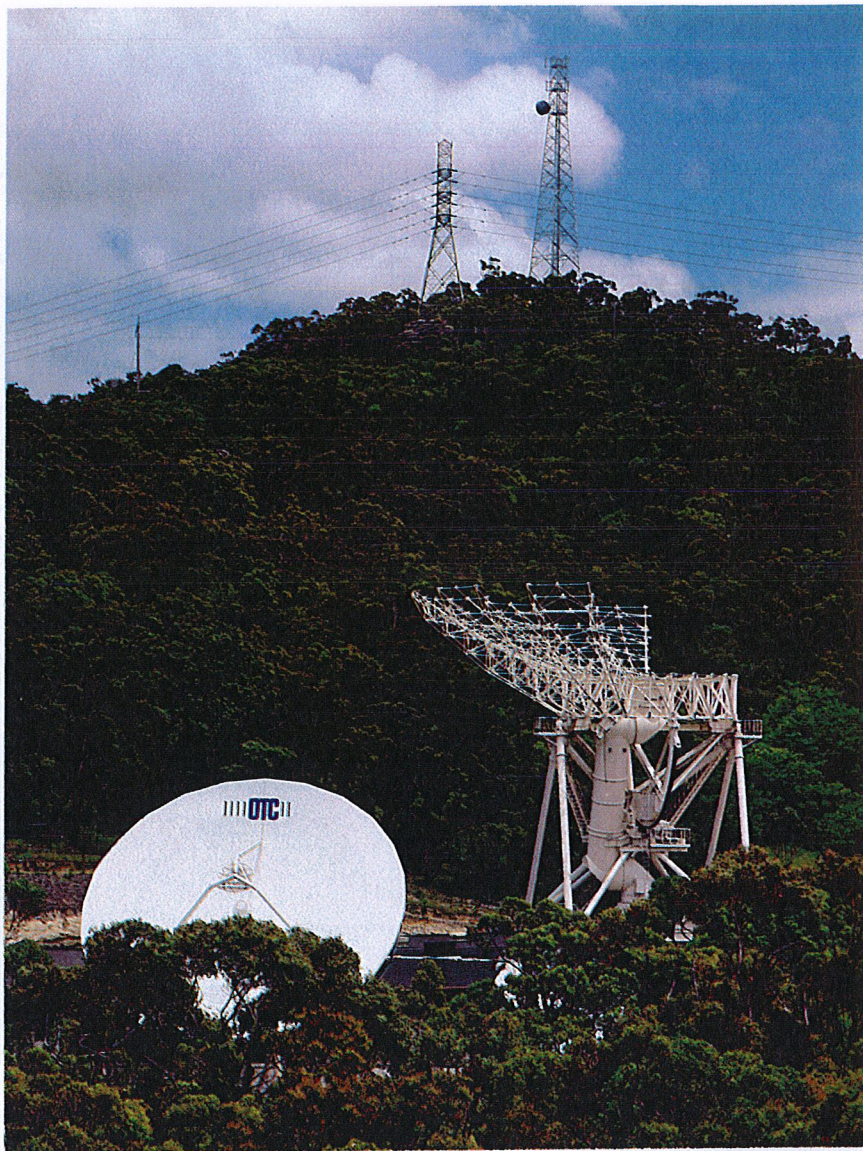
Hi-tech in the bush. The dishes at OTC's Oxford Falls earth station stand out from the greenery of Sydney's north. The microwave dish on the hilltop tower (left) communicates with the Paddington gateway and is linked to the earth station by an optical fibre cable. The incomplete structure is the 32 m Moree dish. In the foreground is the 18 m dish. A view from the Moree dish (opposite), renamed Sydney 2, shows the two smaller dishes flanking Sydney 1, the 18 m dish. The earth station beams signals up to INTELSAT satellites in geostationary orbits above the Pacific Ocean. On the 18 m dish, technical officer Nick Palavic prepares to enter the feed housing. Inside (inset), he checks the feed device that transmits and receives signals through the dish.
